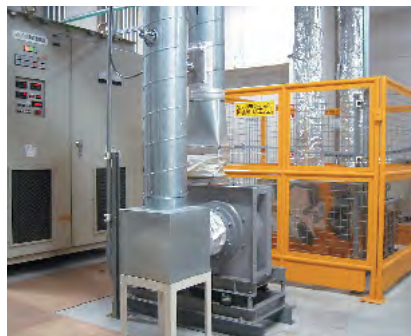
VOC decomposition equipment using atmospheric pressure plasma
