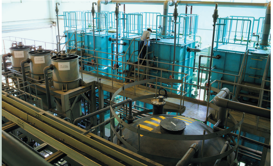
Canon developed a new closed recycling system for processing, purifying, and reusing water and introduced it in Zhuhai, China.
