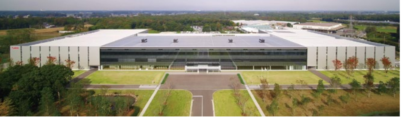
The Canon Eco Technology Park (Ibaraki Prefecture, Japan) was opened in 2018 as a hub for the Canon Group's environmental activities.
