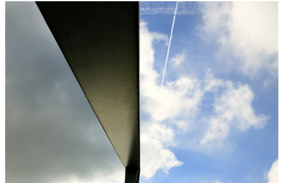
Second Scheldt Bridge, Temse, Belgium (2013)
