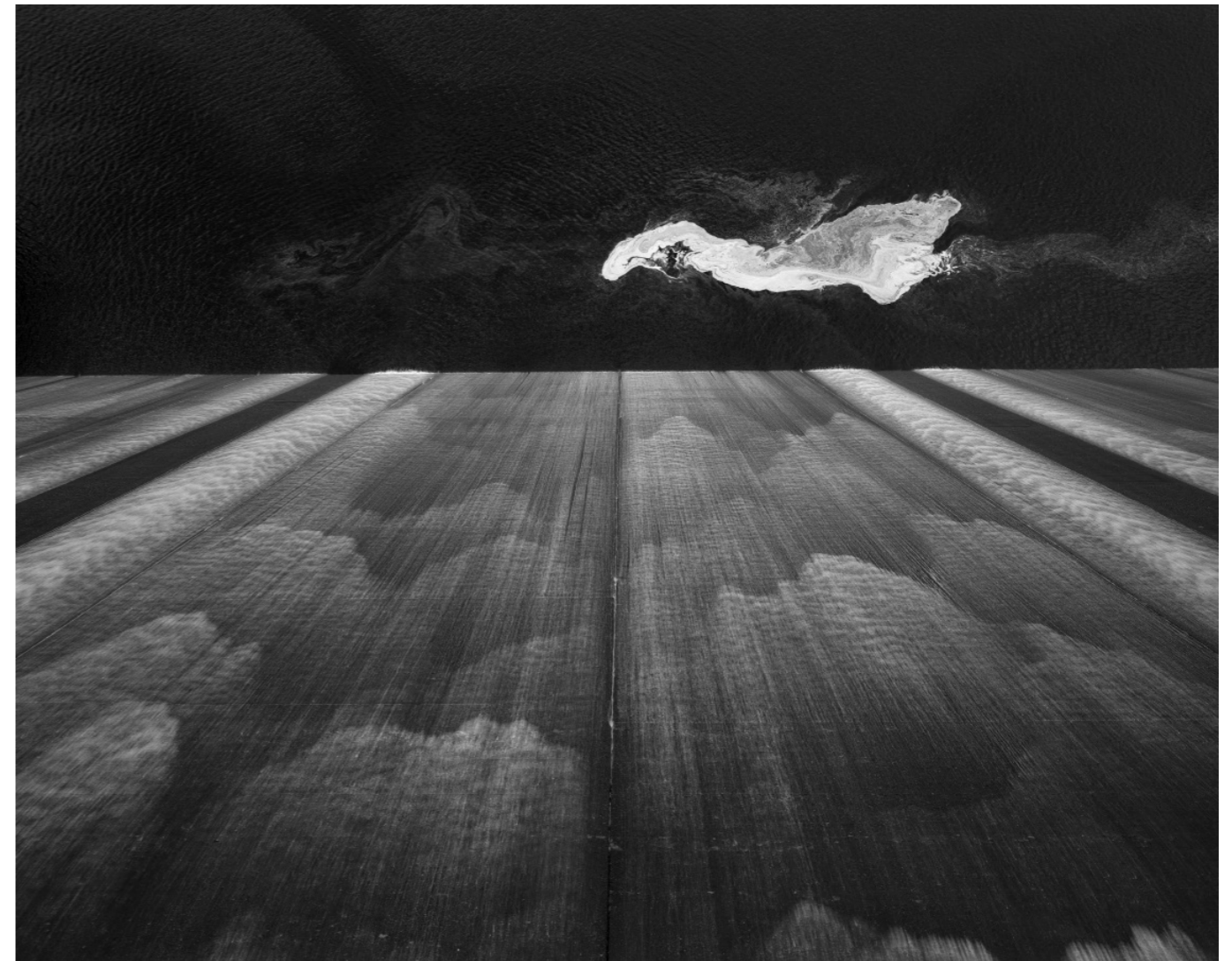
Grand Coulee Dam, Douglas County, WA (1996)
