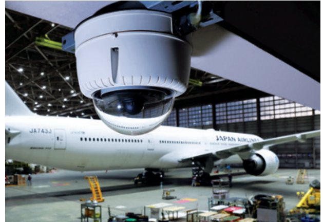
Network cameras are used in various locations
