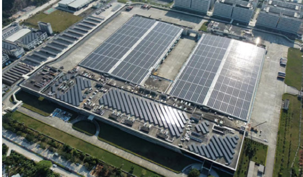
Solar panels installed at Canon Zhongshan Business Machines in China
