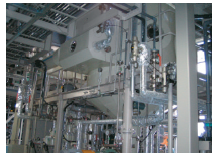
Condenser (Oita Plant of Oita Canon)
