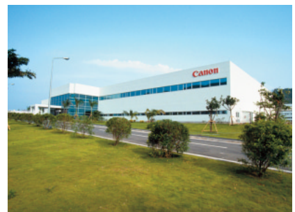
Zero landfill waste achieved at Canon Zhuhai, Inc.
