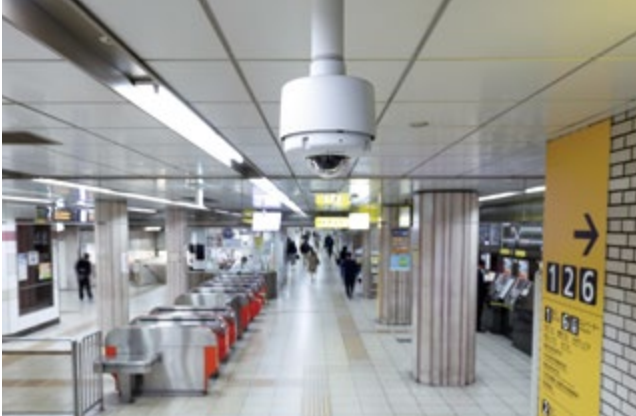
The network cameras are utilized at Akasaka Station. (Fukuoka, Japan)
