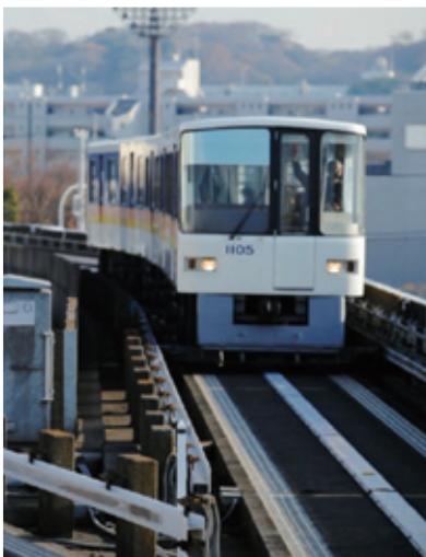
The Yokohama City Seaside Line
