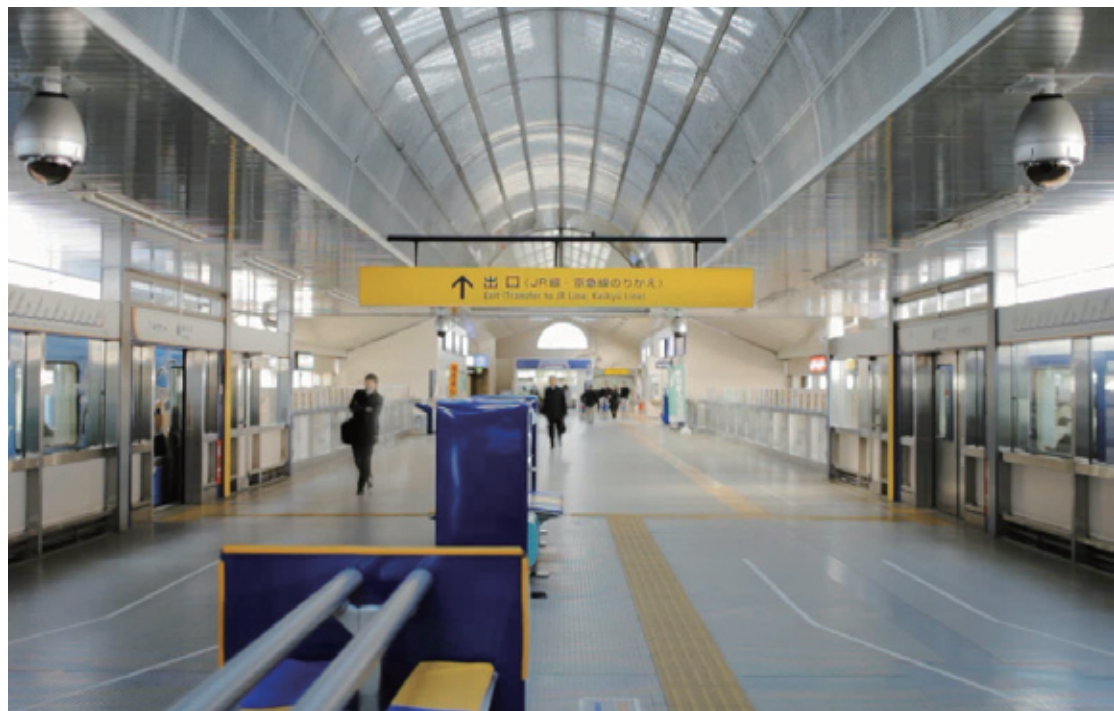
Station platform with network cameras
