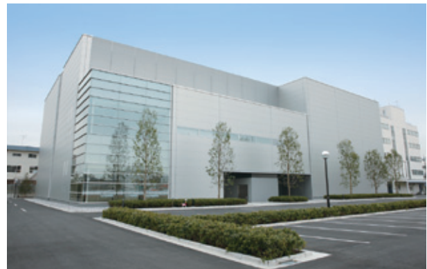
Tamagawa Testing Laboratory
