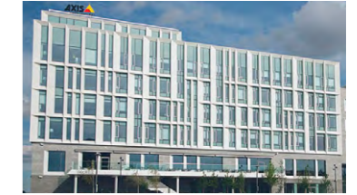
Axis's new headquarters building in Lund, Sweden, meeting the "Excellent" rating under the Swedish version of BREEAM (BREEAM-SE)
