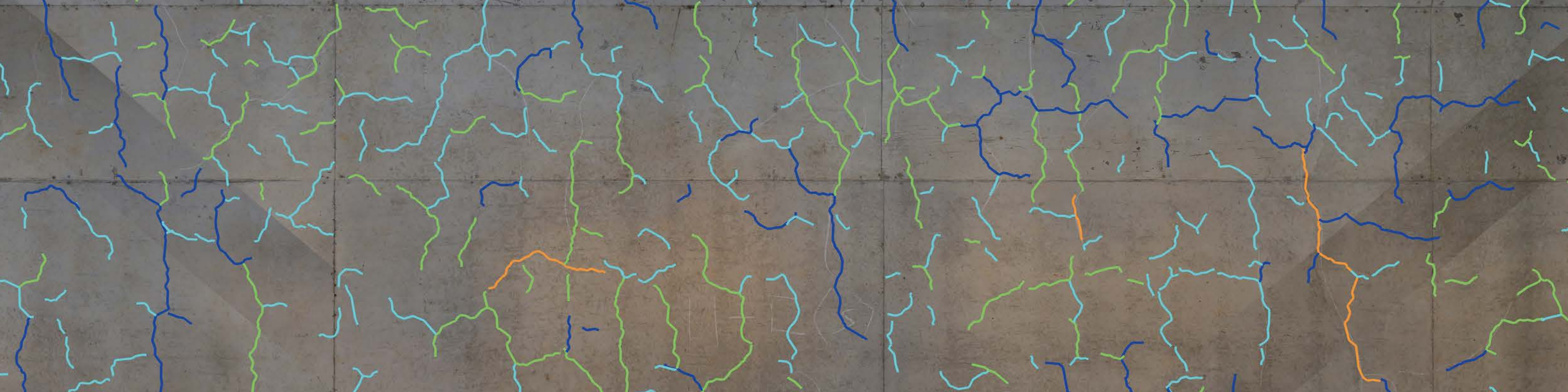
Results of AI crack detection
