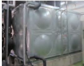
Tank that stores drain water
